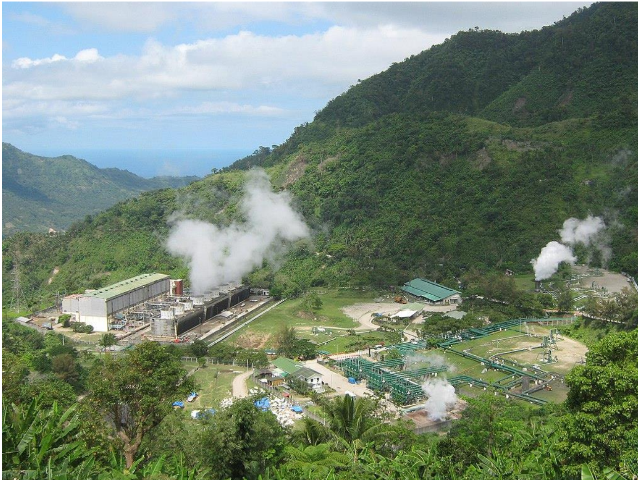
Geothermal power plant in Valencia, Negros Oriental
